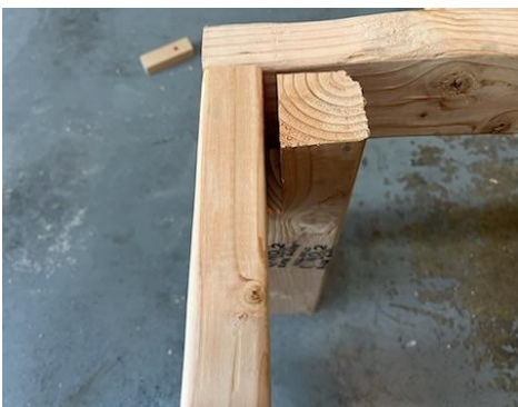
Part of 4x4 is cut away so that it nests with outer frame (see drawn plan for details).
