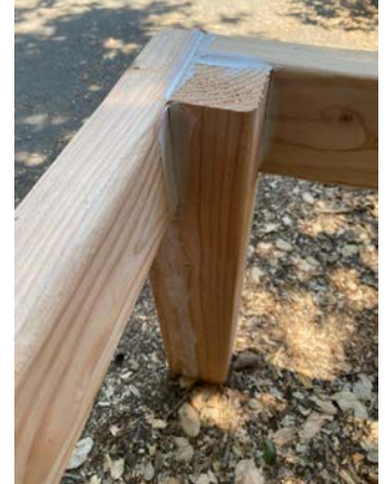
Part of 4x4 is cut away so that it nests with outer frame (see drawn plan for details).
